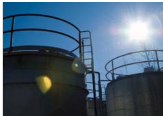
Mixing tanks at LioChem production site
